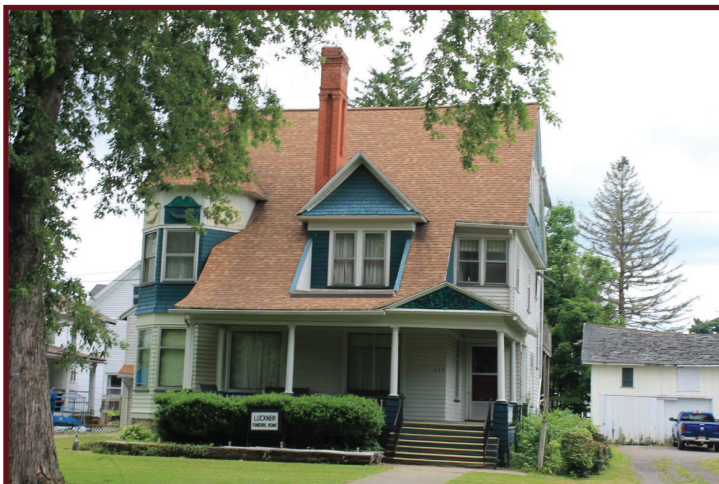
Image 19: House in Waverly Source: Thoma Development Consultants
