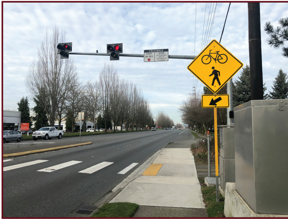
Image 27: Example of a HAWK crosswalk system Source: Thoma Development Consultants
